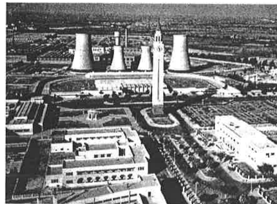
Figure 5. The MSWC in 1949 after the establishment of its clock tower. Source: Courtesy of MSWC.
