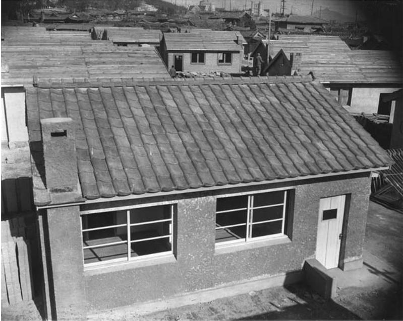
10 A Korean home built with UNKRA funds. Note the smooth exterior, plastered with cement and earth, as well as the tiled roof laid on top of a wood base. Source: UN UNKRA online exhibit S-0526-0350-6, United Nations Archives.
