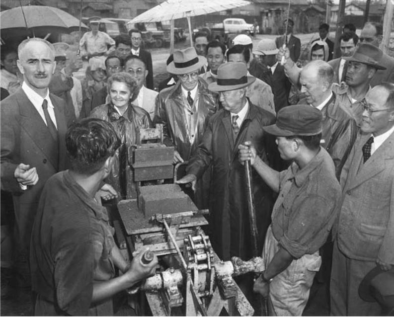
9 President Syngman Rhee and UNKRA head General John Coulter inspecting Landcrete earth-block makers for the 1953–1954 UN-funded housing program. Each home could be built with the unskilled labor of future homeowners, and cost \$750, with roughly half (\$380) going to imported materials. Source: UN UNKRA online exhibit S-0526-0350-5, United Nations Archives.
